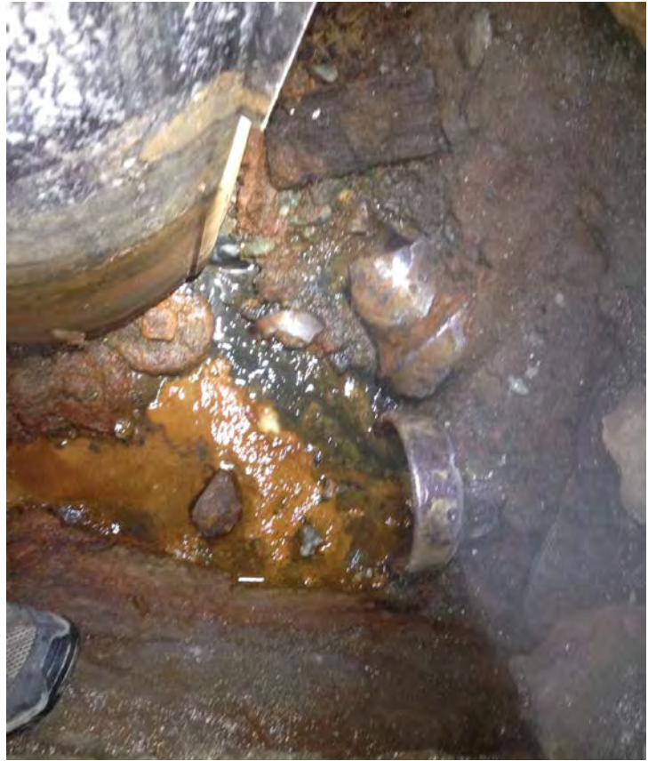
Figure 6. Leaking wastewater pump chamber next to perimeter drain
