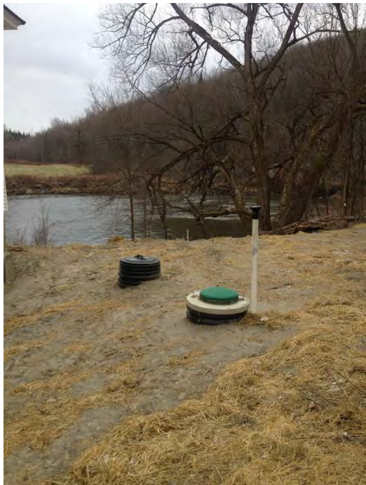
Figure 5. Replacement septic system at the Wolcott Town Hall
