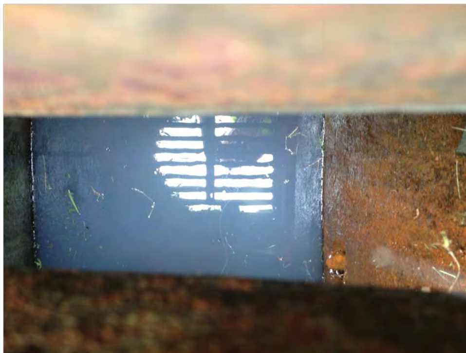
Figure 2. Laundry wastewater present in CB-B in system GA070
